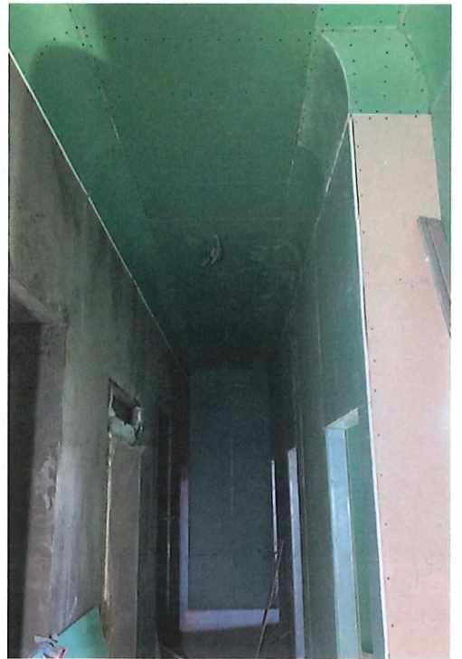
Hallway to future guest rooms.
